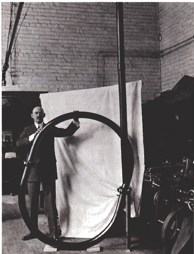
Fig. 1. Robert H. Goddard in 1916 with his circular vacuum chamber. The device was used to demonstrate that the efficiency of a rocket fired in a vacuum was greater than when fired in air. In use, the rocket nozzle was positioned at the top of the vertical tube. The circular portion reduced the rebound of exhaust gases. Photograph courtesy of Goddard Collection, Clark University.
