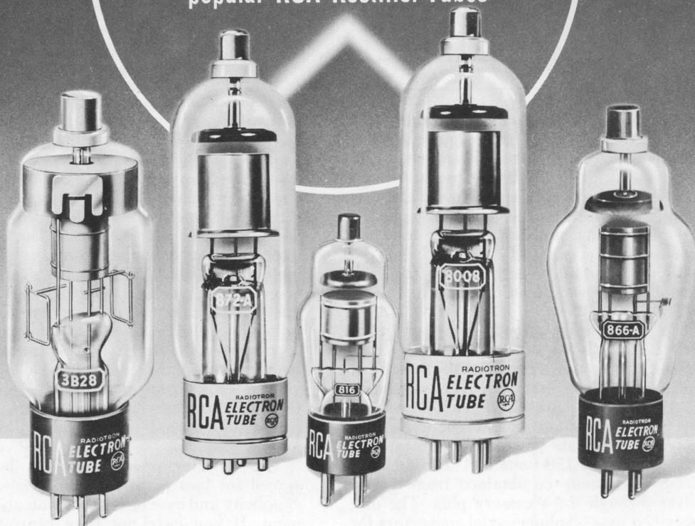
In accordance with RCA's continued policy to provide the radio amateur with the highest performance tubes consistent with the best engineering practice known, every rectifier tube shown here is now designed and built with the new, improved coated filament—N-85-R!
